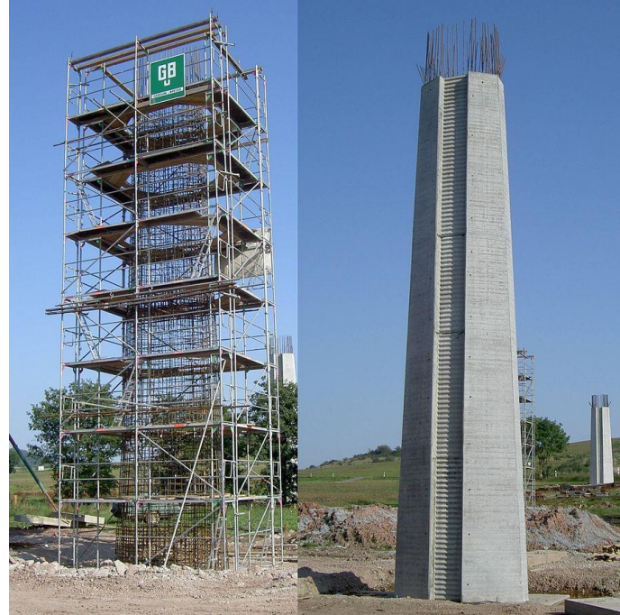
Leg of Talbrücke Brunn during construction CC BY-SA 3.0, Florian.Arnd and Störfix
