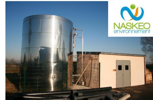
Industrial PROVEO process (50 m 3 ) For dairy effluents
